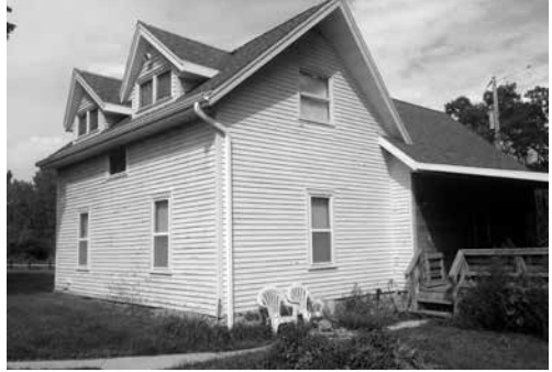
1.6. Recent photograph of the Martin family's home in Ixonia Township. As with the Carlin home, the site agrees with early plat maps and the foundation is consistent with a home constructed in the mid-1800s.
