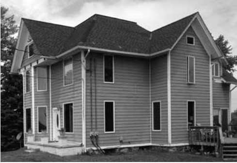
1.5. Recent photograph of the Carlin family's home in Ixonia Township. The site of this home agrees with the site identified on plat maps from the mid-1800s. In addition, close examination of the foundation of the home reveals that it was constructed with fieldstone, making it likely that the home was built in the mid-1800s, when the Carlins lived there.
