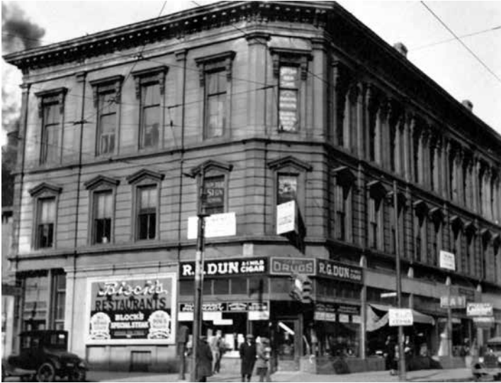
6.1. Central Hall Building (22nd Street and Wabash Avenue), where Martin had his first office, late 1800s.
